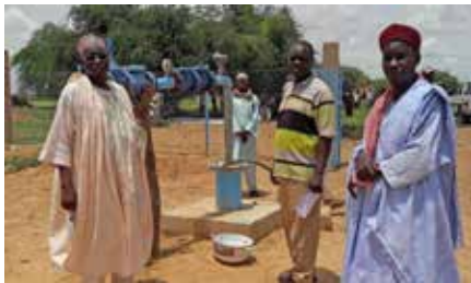
Water supply in the Diffa region (Niger)
