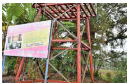
Renovation of water tanks in Nicaragua
