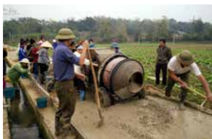
Road construction in the municipality of Duc Xuan, Cao Bang
