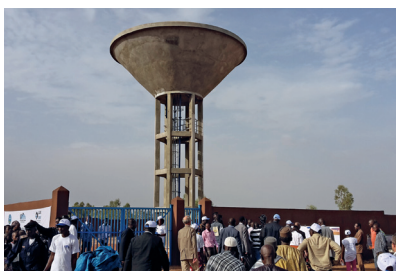
Mali - Inauguration of the new drinking water supply at Sénou. This new infrastructure, financed by the Grand Duchy of Luxembourg, will produce two million litres every day, supplying the drinking water needs of 40 000 people
