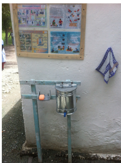
Tajikistan - Patríp project in Dushanbe, Tajikistan: entrance to communal sanitary facilities
