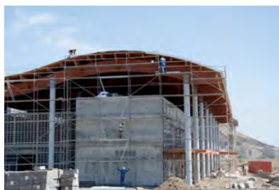
Cabo Verde - Construction of the ERMI renewable energy vocational training centre
