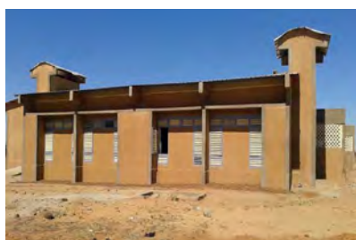
Niger - Bricklaying training centre
