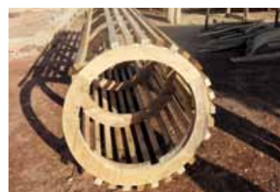
Water tower under construction in Ségou
