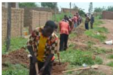
Mali - Installing drainage
